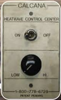
Modulation Control Panel
